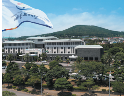
A view of the Overseas Koreans Foundation headquarters building on Jeju Island.
