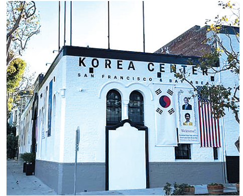
The San Francisco Korean American Community Center, which was renovated for the first time in 100 years
